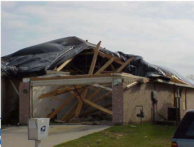
FIG. 9 - WIND - BEHAVIOR ON GARAGE DOOR TRACK ASSEMBLY
