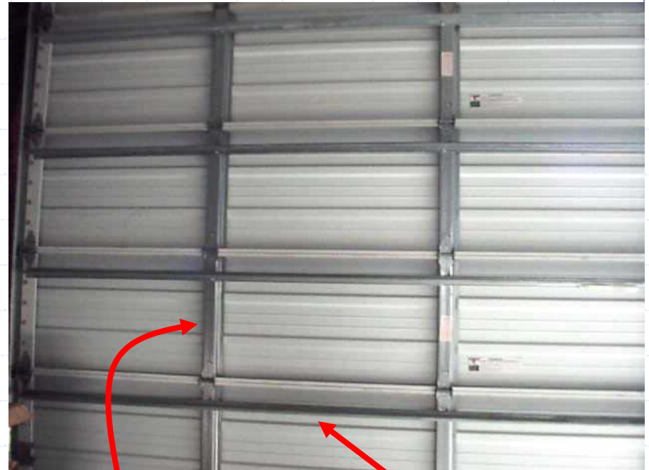
Vertical reinforcement in door design
