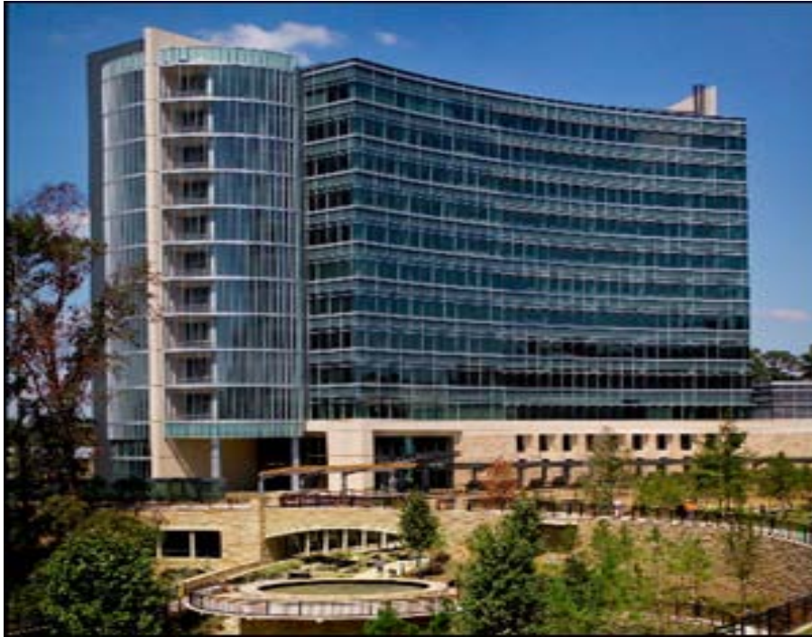
The exterior of the new "Arlen Specter Headquarters and Emergency Operations Center", otherwise known as Building 21, located on CDC's Roybal campus in Atlanta, Georgia. (Photo by James Gathany)
