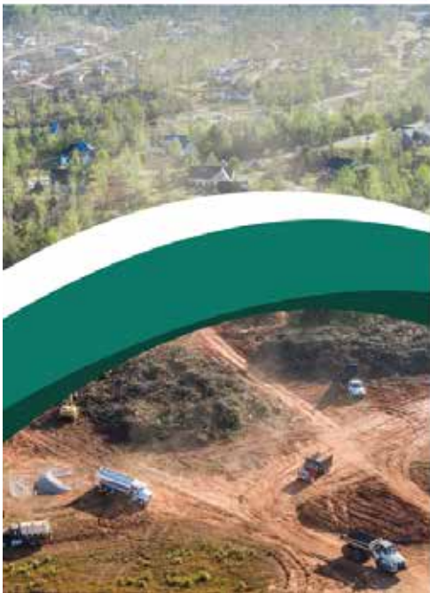
Disaster Debris Removal
