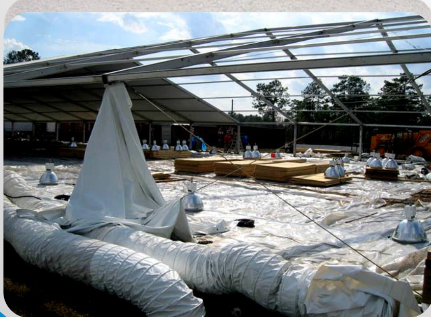
Long Span Structures
